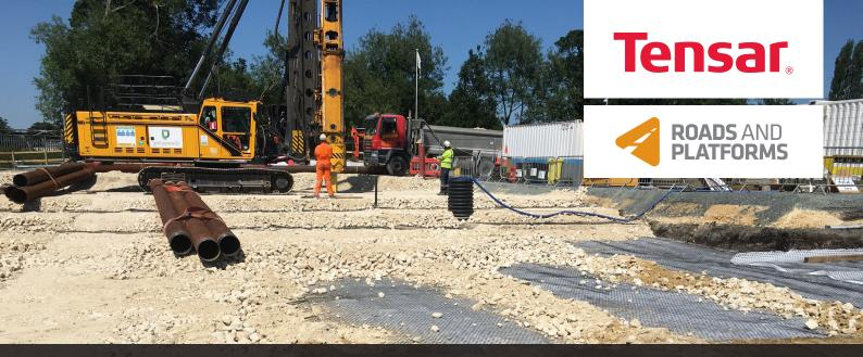
Three new settlement tanks were supported by driven precast piles, installed through very weak clays and founded in the underlying chalk bedrock.
