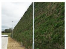
**TensarTech GreenSlope** is designed for up to 70° slopes, maximising development space.
