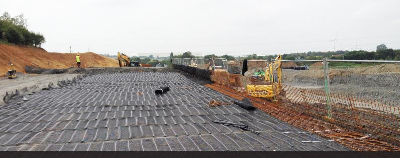
Tensar uniaxial geogrids reinforce the fill used to build the 15.5m high earth bund.
