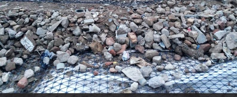
TriAx incorporated under both the capping and sub-base layers delivered a cost-effective design that reduced pavement thickness and mitigated differential settlement.
