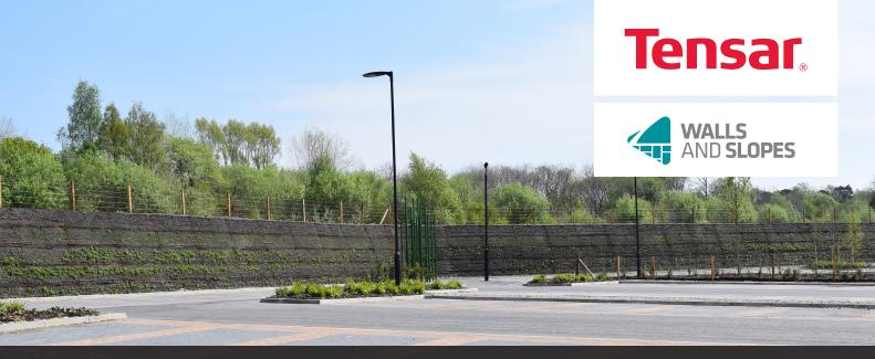
Tensar's TensarTech GreenSlope system was used to build the 70° slope, maximising car parking space, with a natural, vegetated finish helping it to blend into the surrounding landscape.
